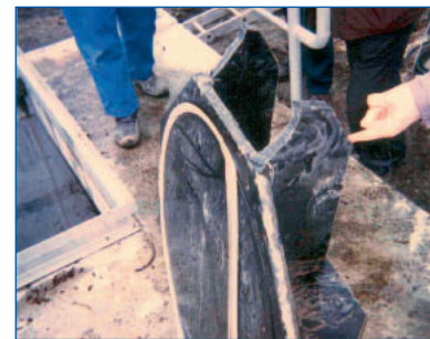
Fig. 1-c: DN 800 check valve following a pressure surge in the discharge pipe
