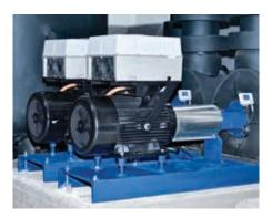
2 Etanorm PumpDrive pumps for continuous operation with high-efficiency KSB SuPremE<sup>®</sup> IE5 motors\*
