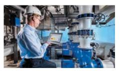
Pump Operation Check with PumpMeter
