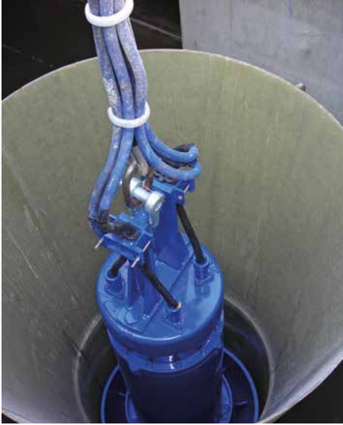
Fig. 86: Lowering an Amacan into the discharge tube
