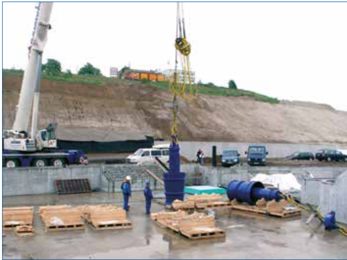
Fig. 2: Installation of a submersible motor pump with a mobile crane
