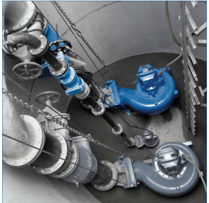
Fig. 52: Vertical valve arrangement in the pump sump
