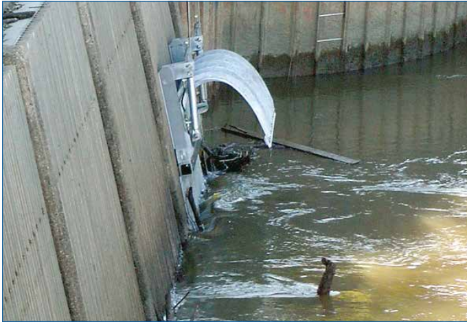
Fig. 84: Screen with automatic cleaning system
