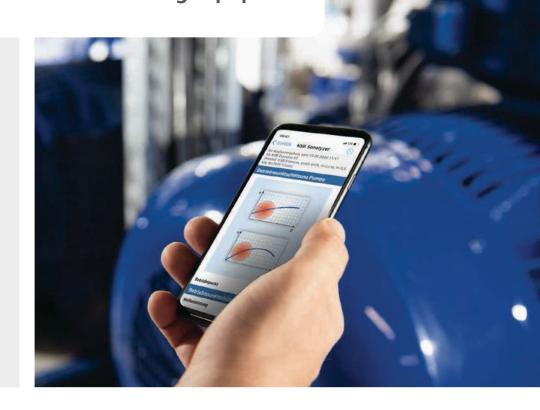
First of all, select your pump type in the app and enter its data, which you can find on the name plate. Then record your motor's fan noise for 20 seconds. The measurement result shows you whether the operating point of your pump is inside or outside the part-load range. This gives you a direct indication whether energy savings can be made.
