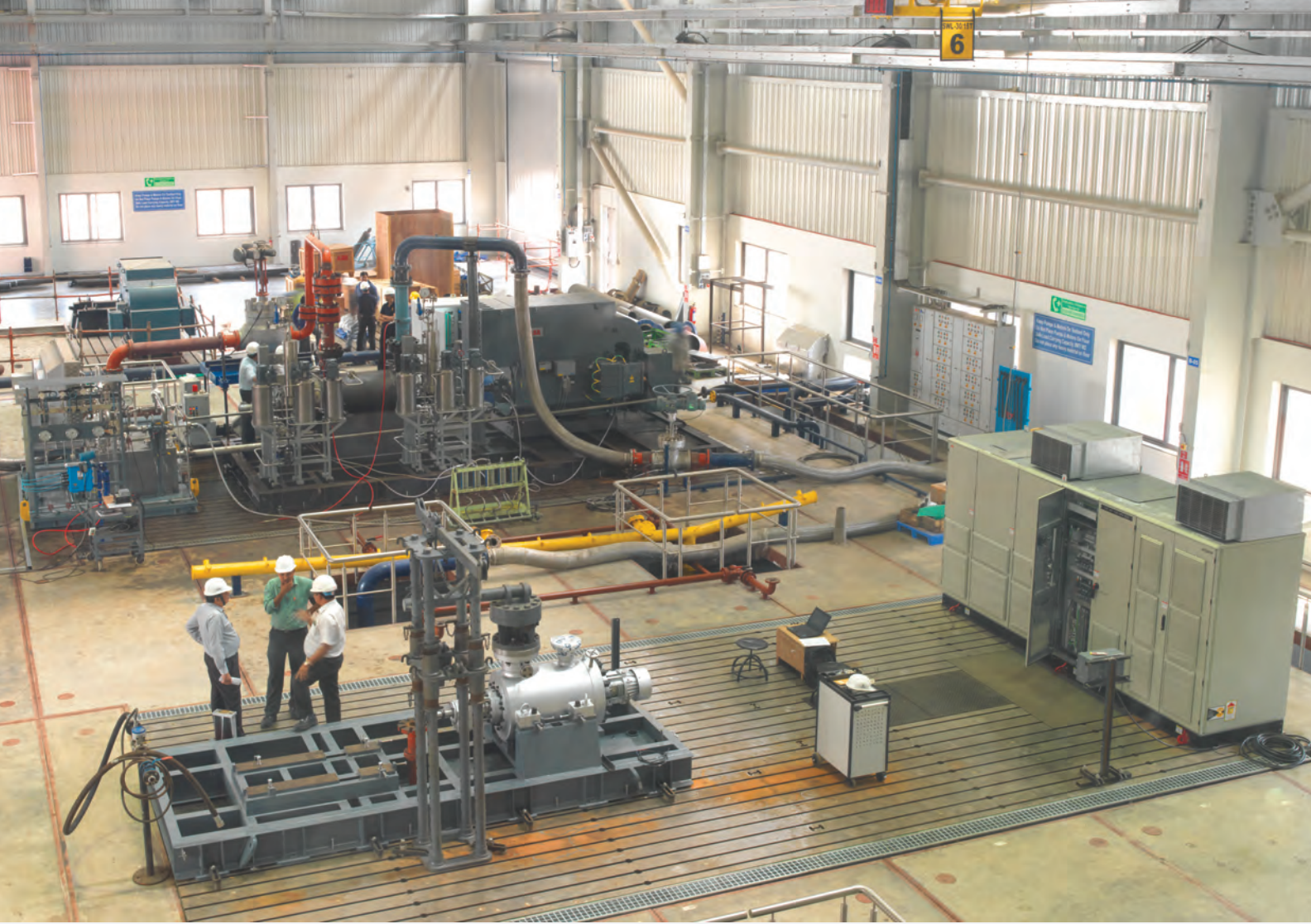
High pressure, multistage barrel casing pumps CHTR 5/9 with motor of 1300 kW were tested at Energy Pumps Division . These pumps will work as main pumps in one of the LPG pipeline projects in India.
