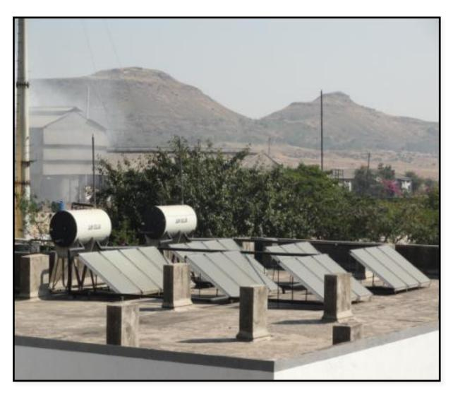
We have installed Solar panel on roof-top of the canteen. The hot water produced is used for various canteen purposes.
