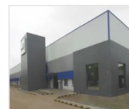
Foundry Division, Vambori
