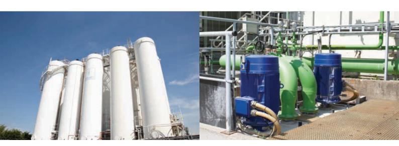
The measurements conducted by KSB Service GmbH showed that the tubular casing pumps installed in the cooling water circuit were considerably oversized for the actual load profile. Searching for energy-optimised replacements for the two old pumps, KSB's engineers compared several design variants of vertical volute casing pumps. They found that volute casing
