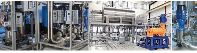
Equipped with PumpDrive speed control and the PumpMeter monitoring system, the Movitec pumps supplied by KSB ensure constant pressure and provide the desired volume of water. The motor-mounted PumpDrive version replaces complex control cabinet solutions. The "Plug & Run" system offers quick and easy commissioning. In addition, all pump, PumpDrive and PumpMeter parameters are factory-set, which means the pump's characteristic curve is already stored in PumpDrive and PumpMeter.
