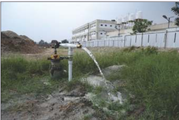
Installation of bore well
