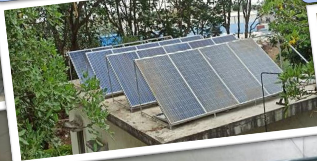
Stand alone Solar energy for ETP/STP Pumps
