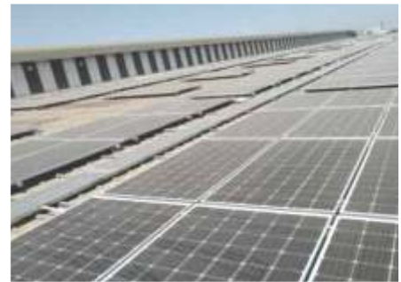
Installation of Solar panel
