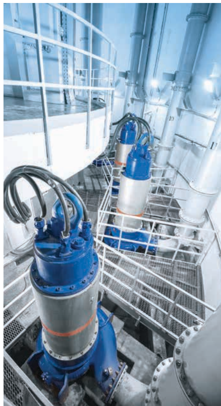
Waste water pumping station St. Petersburg, Russia: With 19 Amarex KRT pumps including control systems and frequency inverters KSB contributes to the continuous treatment of up to 98 % of today's waste water from the multi-million metropolis at the Baltic Sea.
