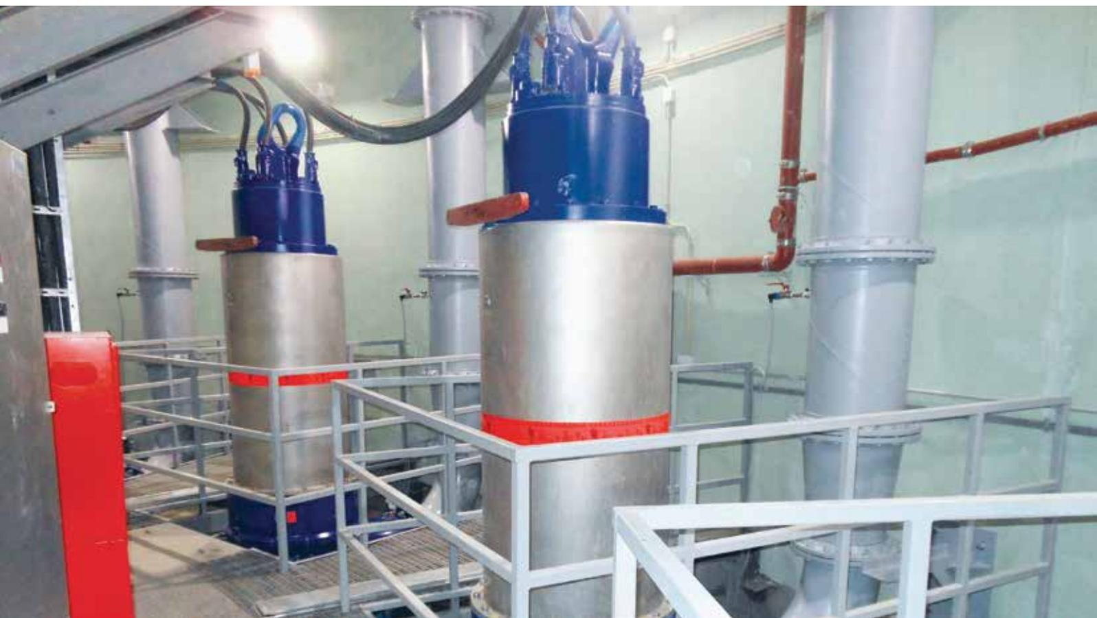
Designed with non-clogging impellers and large free passages, wastewater pumps from the KSB Amarex KRT series ensure efficient operation - even when handling fluids with a high solids content, optimized for every type of wastewater, specially protected cable entry, coupled with sensors trigger a warning in the event of overheating or ingress of moisture.
