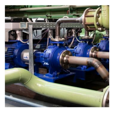
With a wide choice of materials and seals for a large variety of demanding fluids, Etanorm pumps offer solutions for many applications. In Indonesia, KSB Etanorm are in use for various applications such as industry, buildings, energy, clean water supply, distribution, utility, transfer, desalination, fire-fighting systems, cooling water/chiller systems, and other applications.
