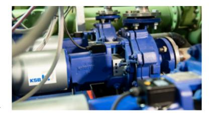
KSB Etanorm is one of the standardized water pumps (to EN 733) of the Eta pump family. Its reliability and economical operation are what make the Etanorm pump a popular choice for various applications. When it comes to energy efficiency, KSB always goes the extra mile. The understandable demand to save energy has greatly influenced our recent development work.
