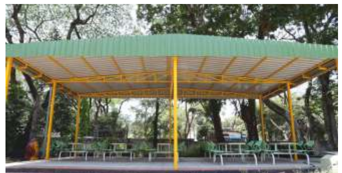
Bal Kalyan Sanstha - Construction of Dining area
