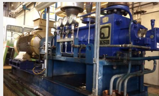
Efficiency improvement of a pump through the installation of the SuPremE motor.
