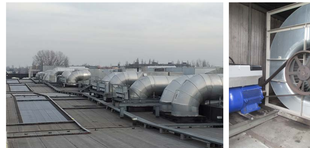
AHUs equipped with SuPremE motors and FlexiMova mm on-board motor converters at Coop Alleanza 3.0 plants
