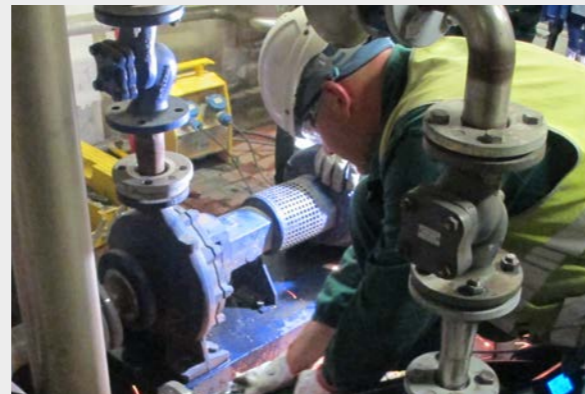
Energy efficiency improvement works at a Galbani plant granting 39% energy savings.
